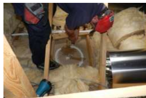
Fig 3 – Avoid dust and cut from above
