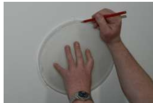
Fig 2 – Mark the ceiling position
