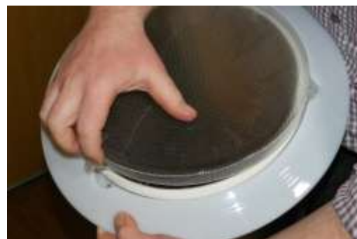
Fig 1 – Use finger pressure to remove the diffuser from the ceiling ring
